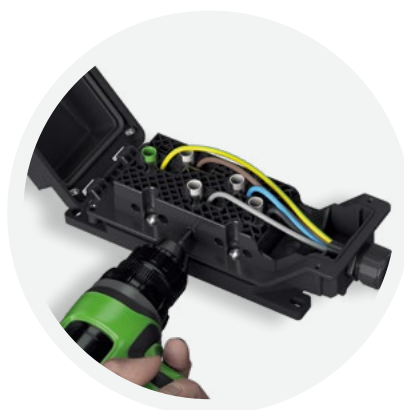
Fastening the wires
