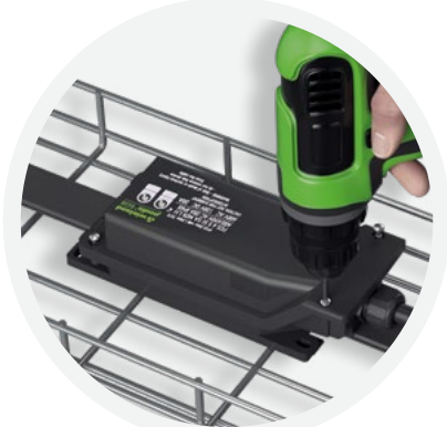
Closing of the housing. Finished!
